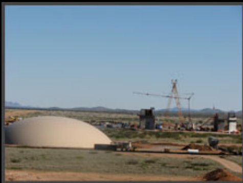
ARFF Dome Construction
