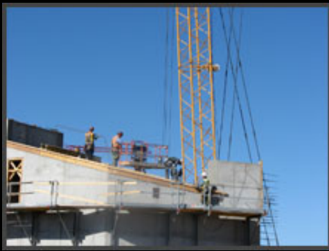
THF Concrete Stair Support Tower Constuction
