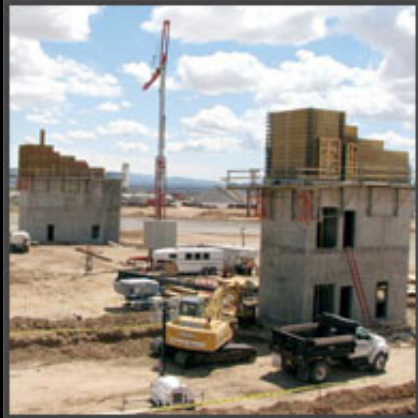
Terminal Hangar Facility Construction
