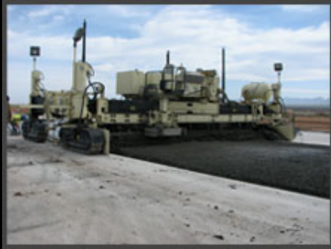
Runway Concrete Leveling Work
